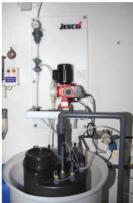
Feeding tank MEMDOS for chlorine dioxide solution dosing
