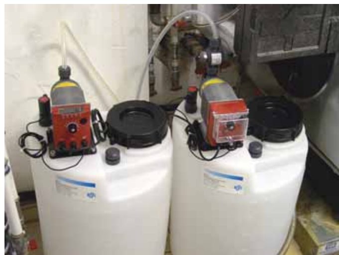
Chemical Feed Systems consisting of Solenoid-driven Diaphragm Dosing Pumps MAGDOS LT and MAGDOS DE, supply tank, level relais, hand mixer, multi-function valve PENTABLOC Figure: www.beste-wasser.de
