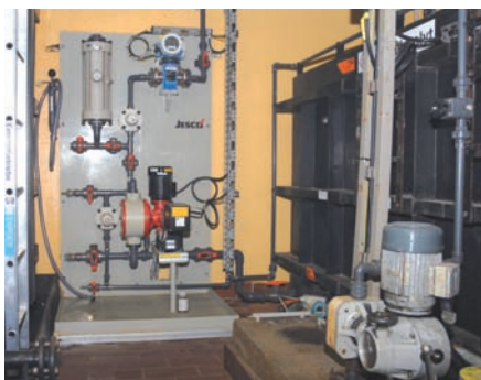
Customer-specific dosing systems as replacement for an installation, that was in operation for almost three decades with Lutz-Jesco pumps
