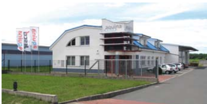
Company building of aquina, s.r.o. in Proßnitz, Czech Republic
