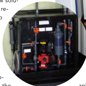
Dosing-container PWT 5.9 with Lutz-Jesco dosing technology
