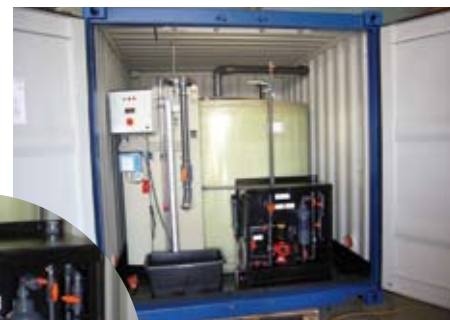
Dosing-container PWT 5.9 with Lutz-Jesco dosing technology
