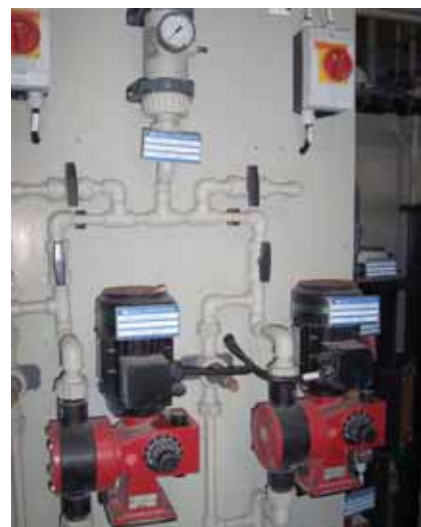
Chemical feed station with MEMDOS diaphragm dosing pumps and a pulsation dampener for the almost pulseless dosing of chemicals.
