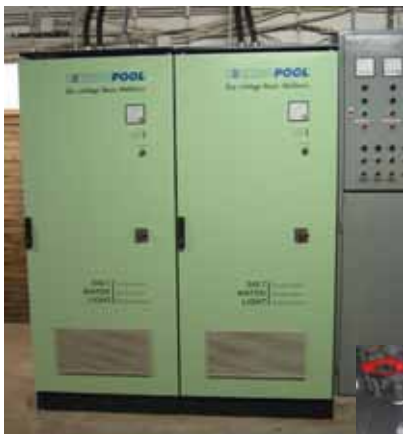
Two Technostar 4000AT saltwater systems with the appropriate electrolysis cells are applied in Obernkirchen.
